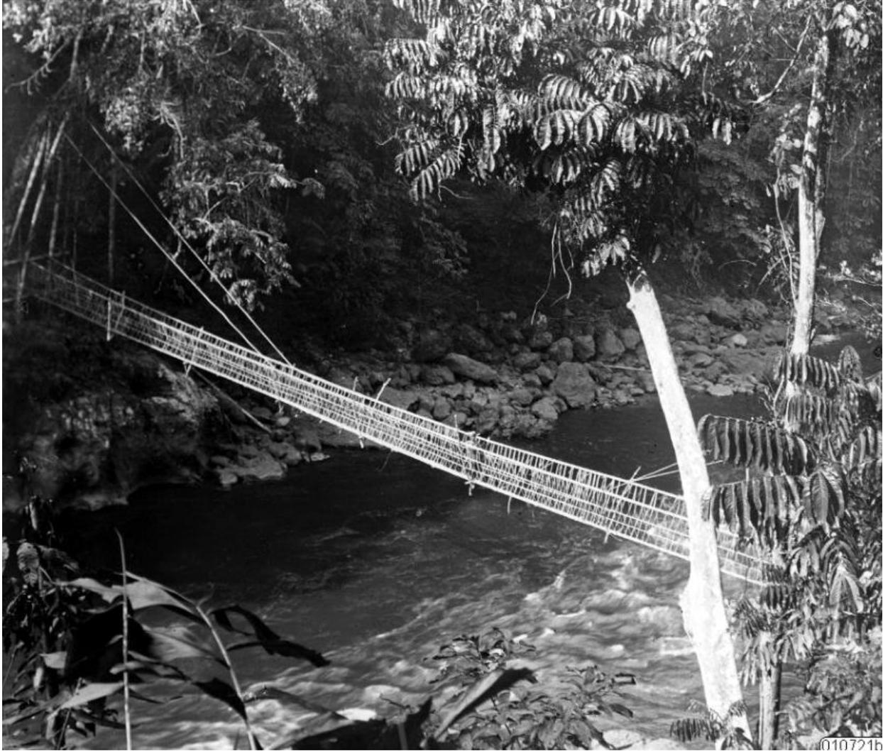
Image 102. The large rattan bridge over the Koro at the former village of Moe. The bridge is 47 m long and hangs approximately 12 m above the water. [Sumber foto.](#)
